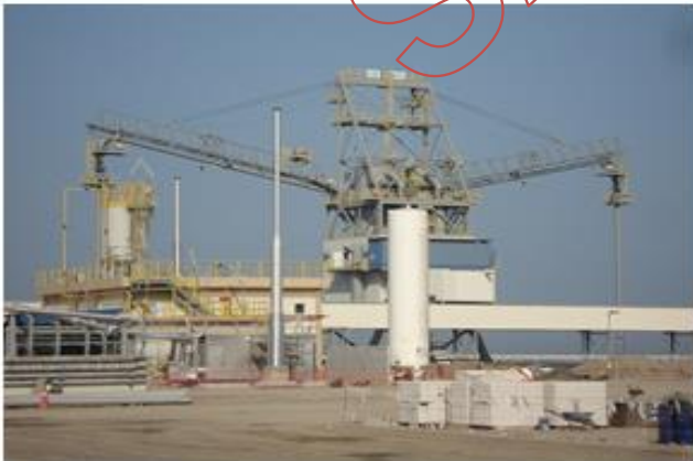
Ship unloader and quay conveyor
