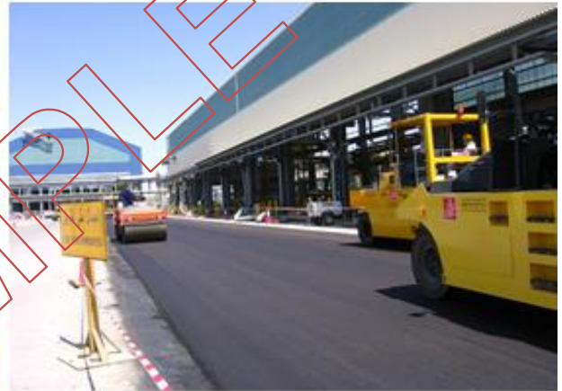
Asphalting outside the Crucible Cleaning Shop
